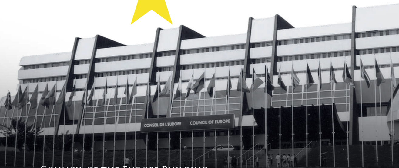
COUNCIL OF THE EUROPE BUILDING
