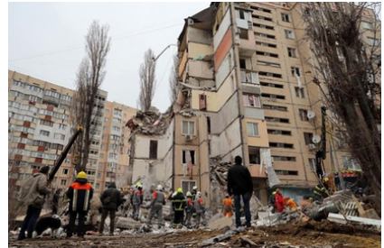
A destroyed house as a result of a Russian missile attack on Odesa on March 2.
